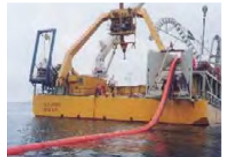
3. The HVAC cable and SeaSerpent being deployed at Havelet Bay.
