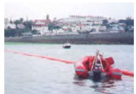
4. Small work boats are used to tow and position the cable.
