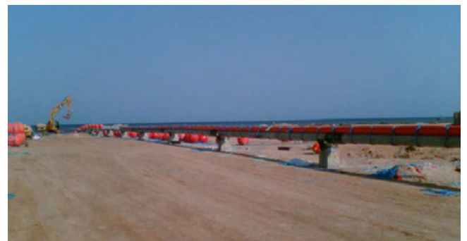
Kraken™ fitted to the Chergui Pipeline, Tunisia, for Petrofac
