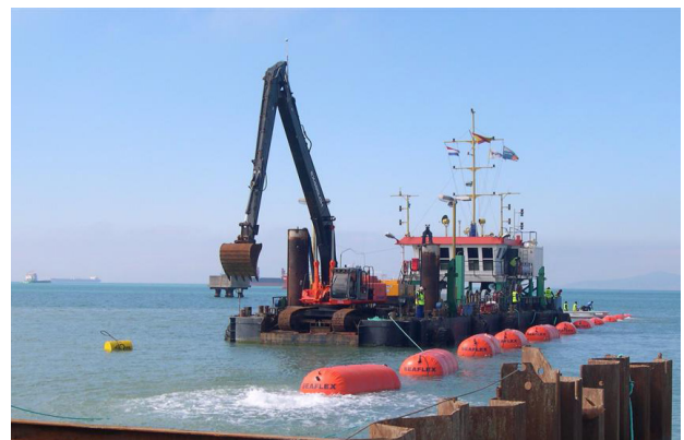
Second String Sinking.
