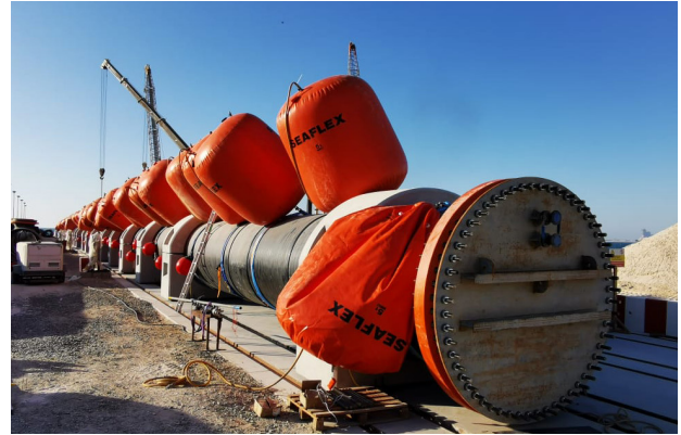
Capped-off HDPE pipe, fitted with deflated Mono Buoyancy Units.
